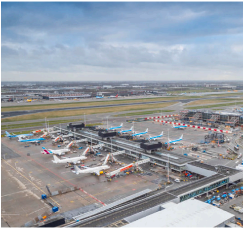
Fig. 4. Aerial view of pier B Chui (2020).
