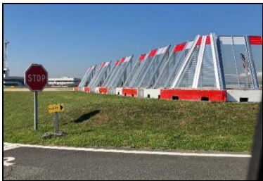
Jet blast hazard mitigation
